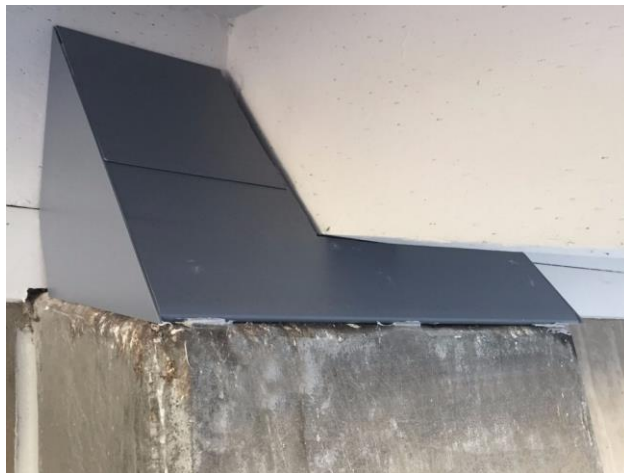
Figure 8. Bird slider for feral pigeon management
