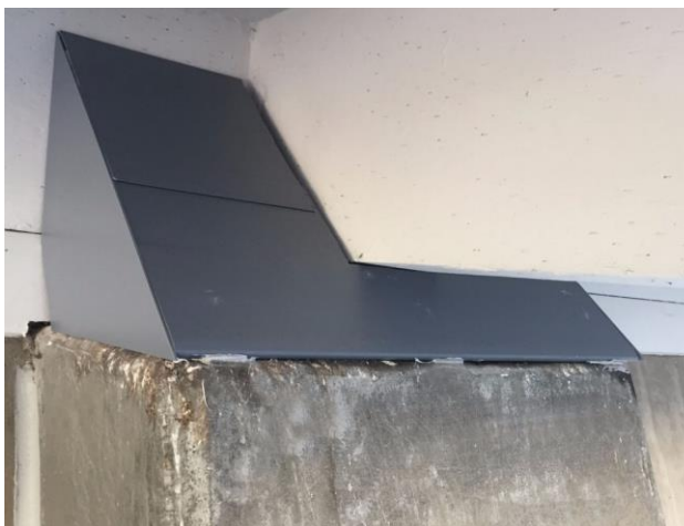
Figure 8. Bird slider for feral pigeon management
